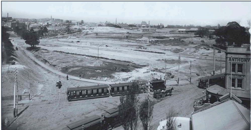
Devonshire Street Cemetery demolition looking towards Chippendale
